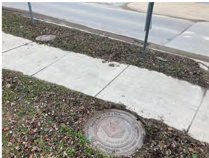
Image 3: Photo of AquaShield Stormwater Treatment Solutions manhole cover. Photo by taken Ira Adolphues .
