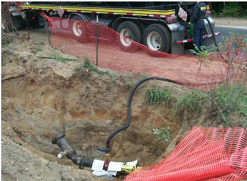
Figure 2. Example Photo of Crude Oil Pipeline Decommissioning
